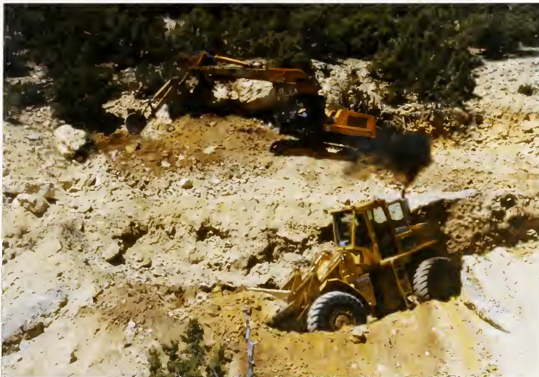
Regrading Waste Dumps Following Pneumatic Backfilling And Preceding Revegetation
